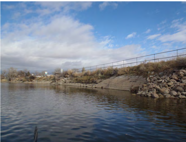
Retaining Wall-Deflector Map-10-080
