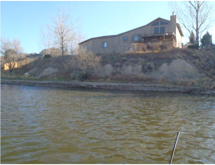
Rock Toe-Pipe Map-2-020
