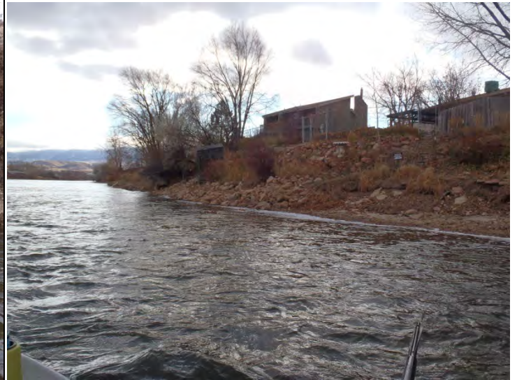
Rip-Rap-Retaining Wall Map-6-059
