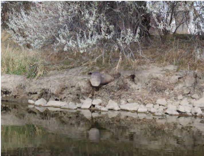
Steel Storm Drain Pipe Map-10-092
