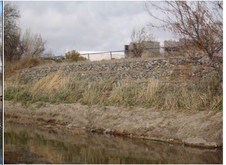
Gabion Wall Map-10-094
